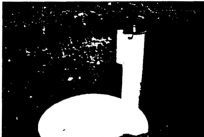
The shelter placed in an excavated area with entrance way attached prior to covering with earth.
